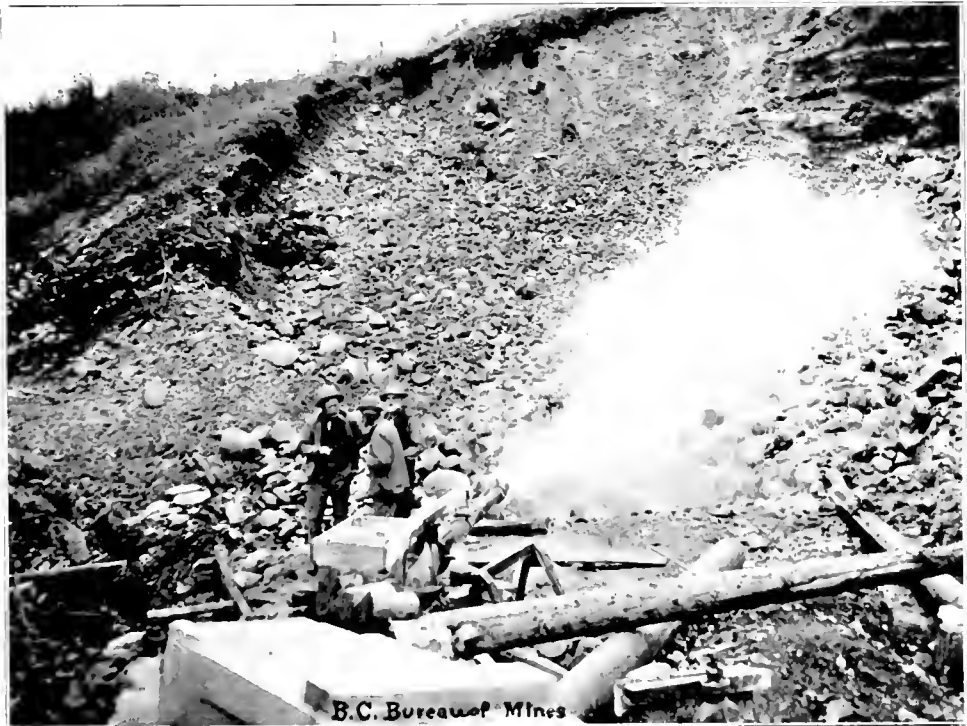
Opening Hydraulic Pit, Boulder Creek Mining Co.
